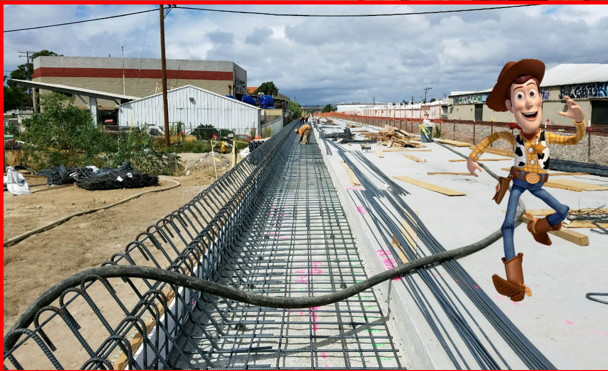
Install waterproofing, ballast retainer and moment slab
