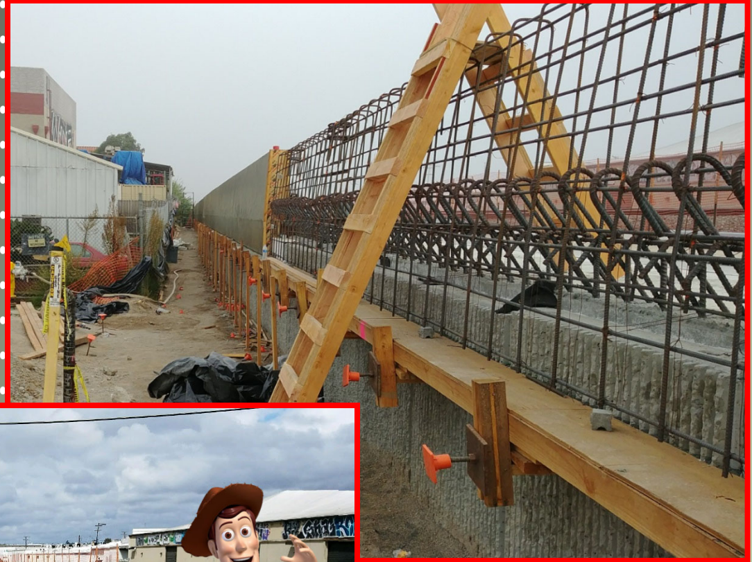
Install waterproofing, ballast retainer and moment slab
